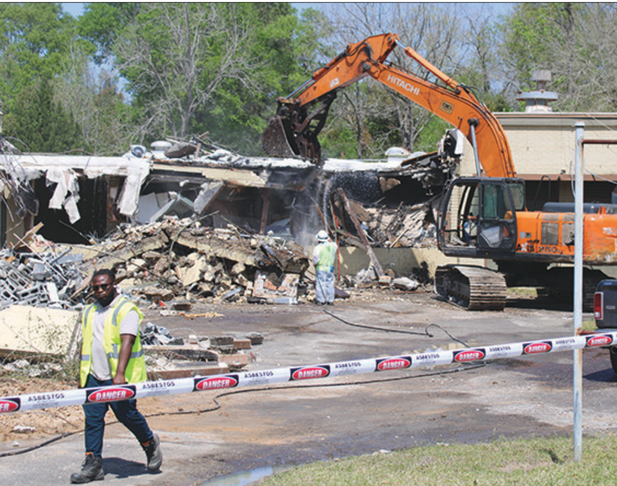
Workmen were seen earlier this week demolishing the former Hardin County hospital building, located near the courthouse on Monroe Street. The area will provide space for a new parking lot, at least for the present, with possible use for another project in the future. The demolishing of the old hospital building is one of several projects now underway in and around the courthouse.
