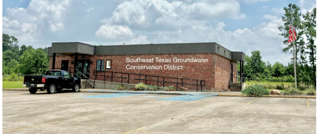
New offices of the Southeast Texas GCD (signage not yet installed – digitally added to photo)
